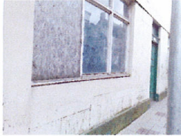
The Old Court House 53 Main St unoccupied more than 10 Years
