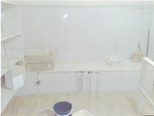
Upper level showing services bulkhead
