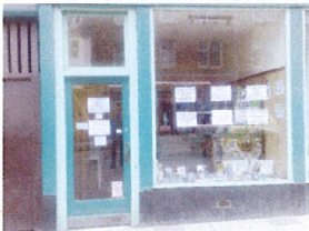
9 Main St unused for retail more than two years
