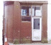
12 Cross St unoccupied more than five years
