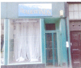
11 Main St unused for retail eighteen months
